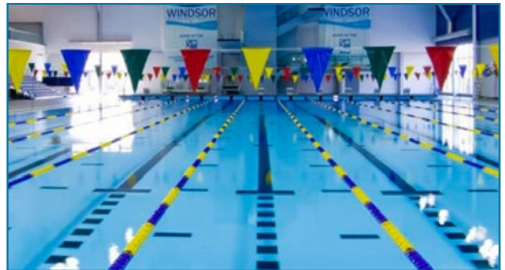
Windsor Aquatic Centre, Canada: Movable floor
